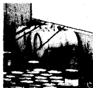
Fuel Tanks For RCN Steam Generator
