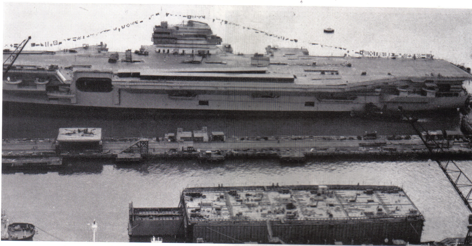
Partially constructed hull of the RANGER is shown in the foreground with the FORRESTAL in the background. The RANGER was placed in the dock vacated by the FORRESTAL for completion.
