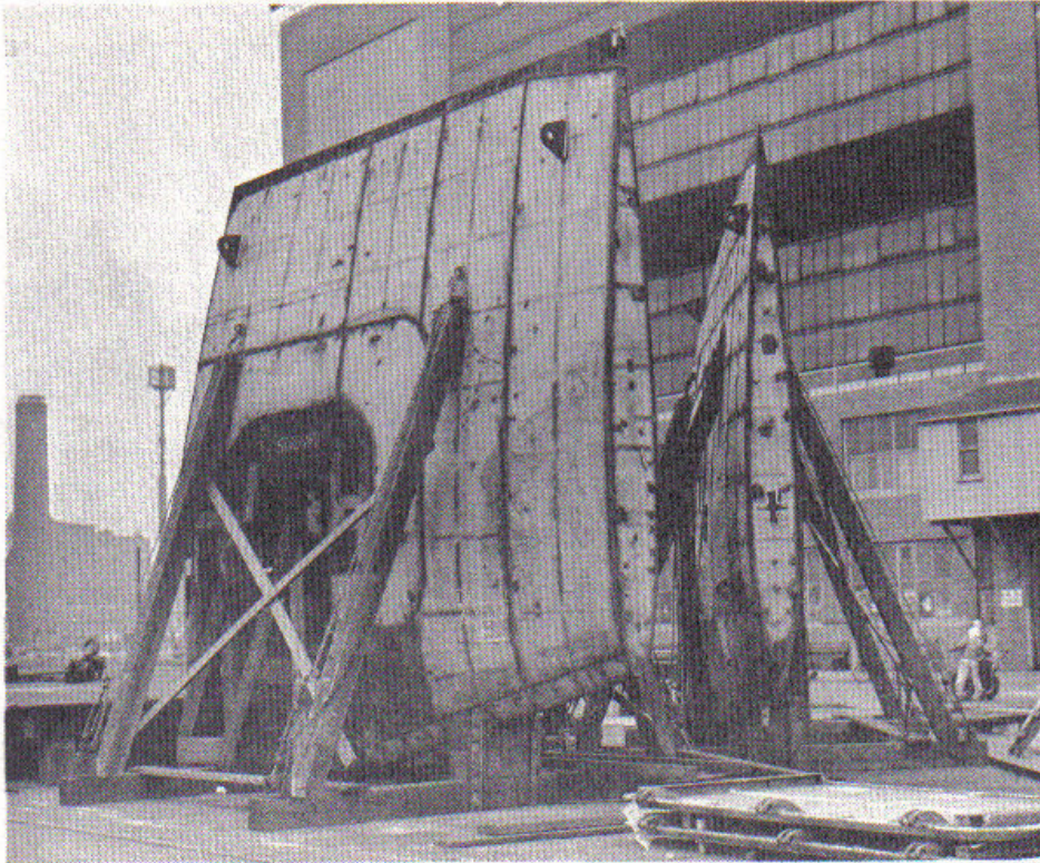
Completed rudders awaiting installation.
