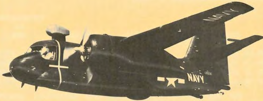
(A) The S2F-2. It featured an enlarged bomb bay and tail surfaces. Only sixty were built during the mid-fifties.
