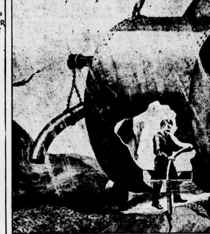
SIMON LAKE'S SUBMARINE WORKING CHAMBER. THE OPERATOR, IN HIP BOOTS AND SURFACE DRESS, GUIDING A SUCTION TUBE IN RECOVERING GOLD FROM THE BOTTOM OF A DEEP RIVER.
