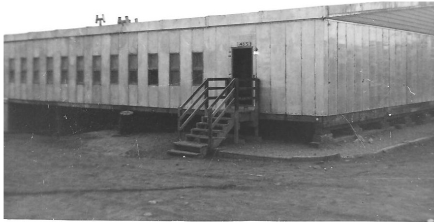
A TYPICAL BARRACKS ATOP THE PERMAFROST AT THULE AIR STATION
