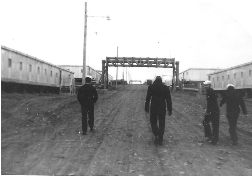
Service lines were provided by trestlework over roads and grounds since Burying lines was impossible in the permafrost at Thule Air Base
