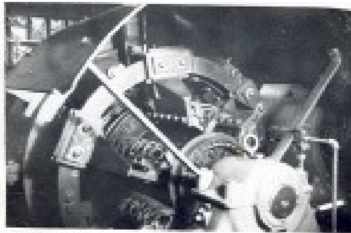
photo shows one of the main electric drive motors which was contaminated with saltwater. the Chinquapin's propulsion system employed two of these motors driving a common gear box which turned the propeller shaft.
