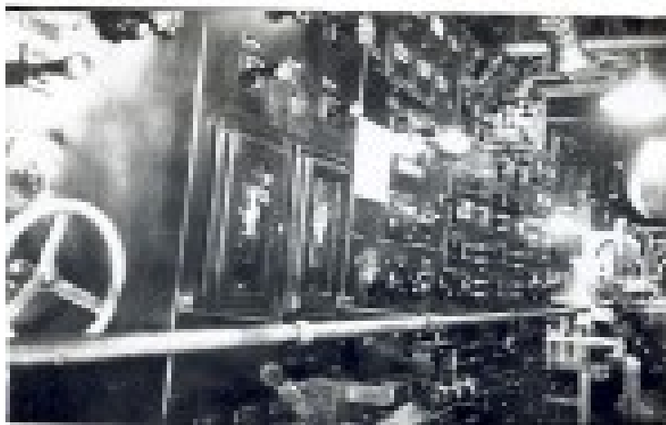
The above photo is of a part of the main electrical switchboard where this writer stood duty watch in the engine room both at sea and in port 4 on 4 off 24/7
