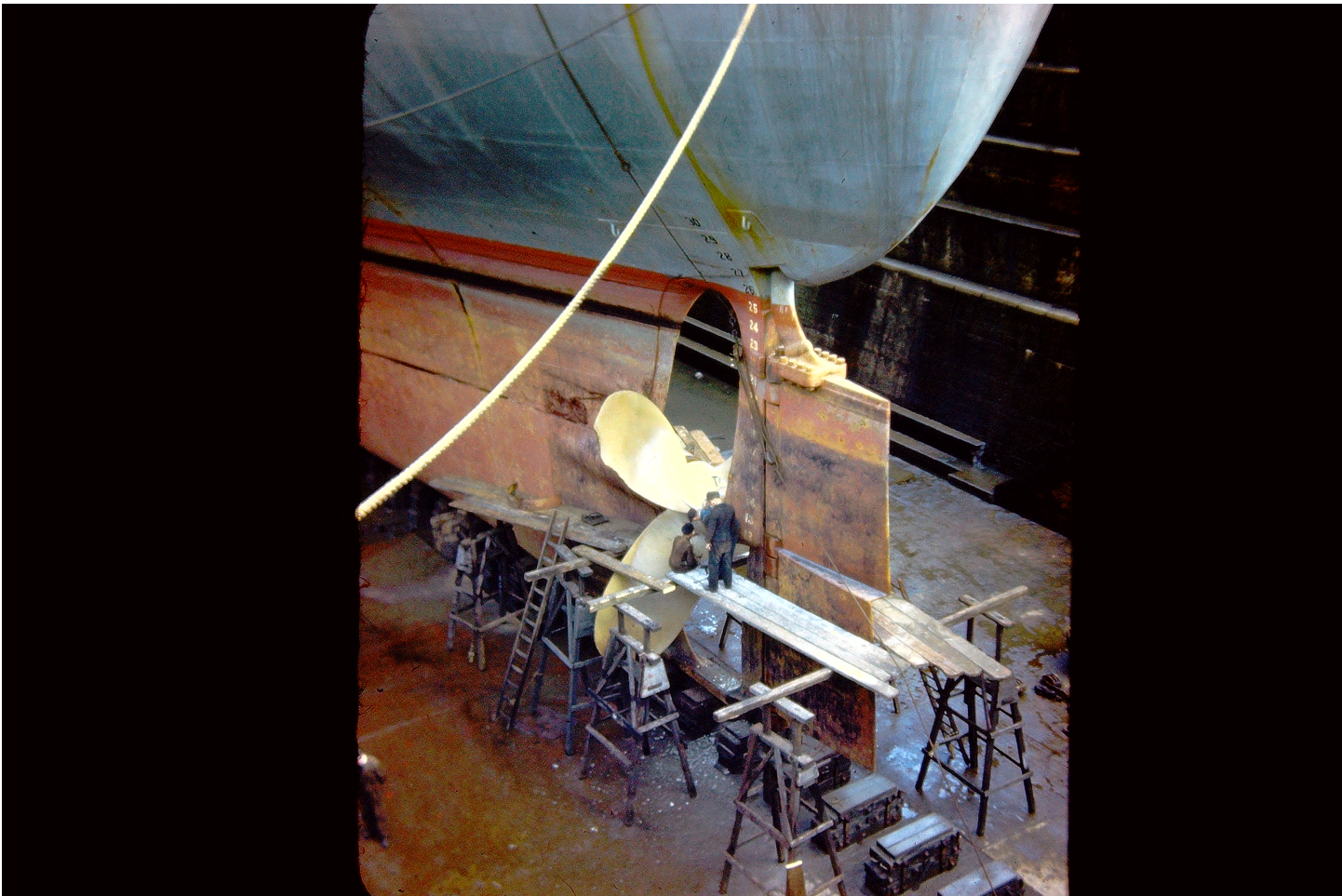
Repairing damaged prop
