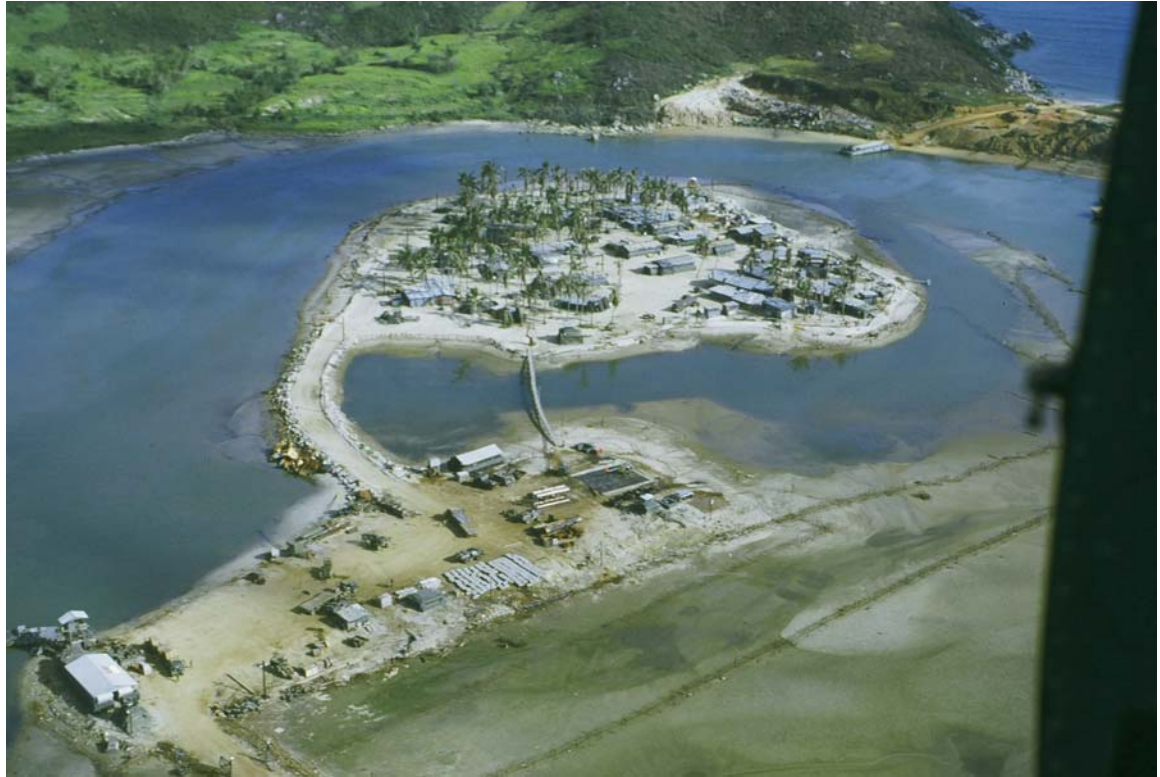
Sa Huynh aerial of boat ramp and main base; 1969.
