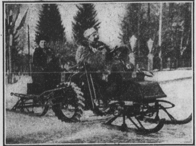
NEW FAD FOR AUTOISTS. A novel Automobile Sleigh, invented by Lieut. Jean de Basse, of the French Army, and which has attained a speed of twenty miles an hour over ordinary good roads.
