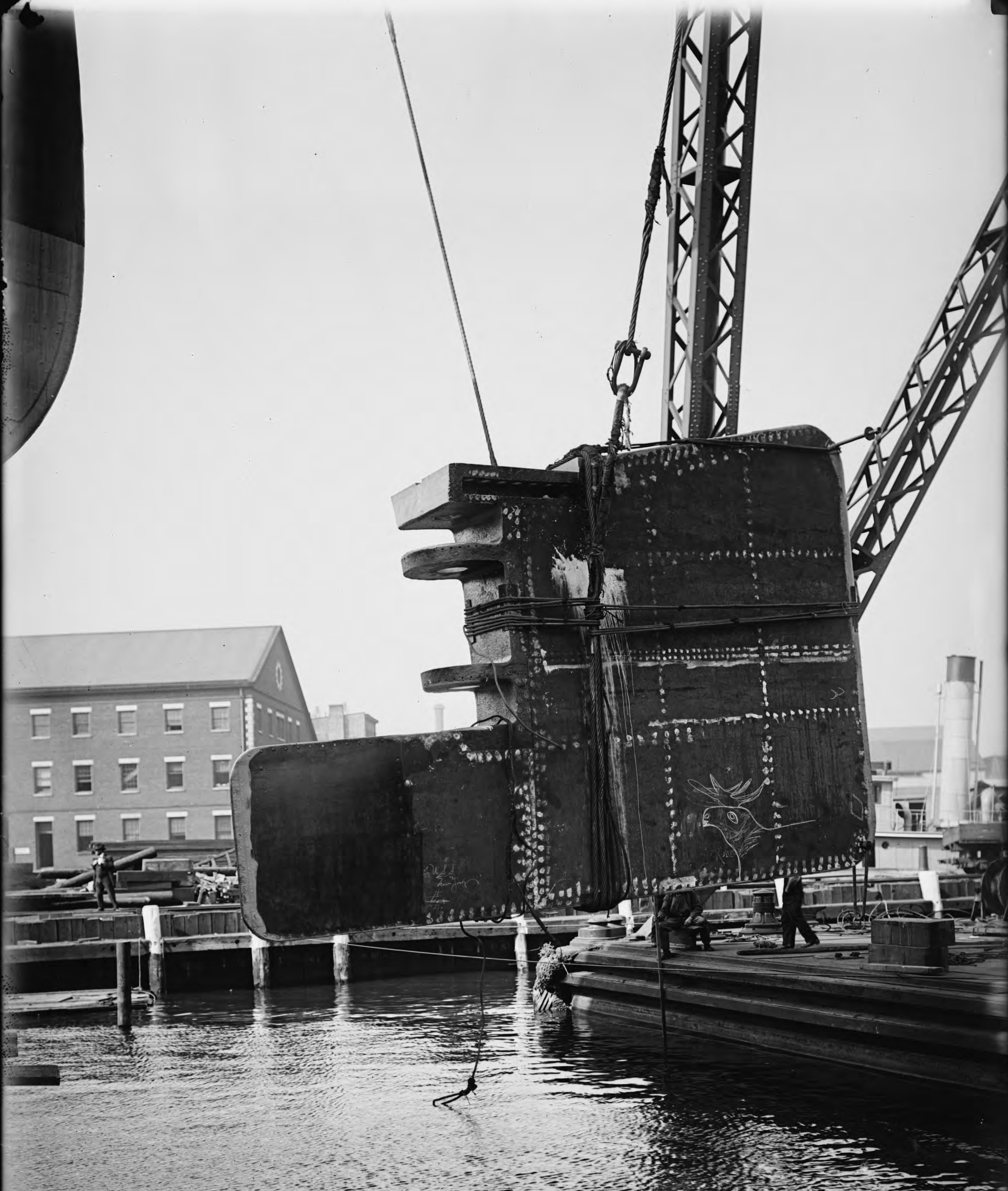
F1003 N6, NAVY YARD, NEW YORK, 10-15-12, U.S.S. NEW YORK, SETTING RUDDER.
