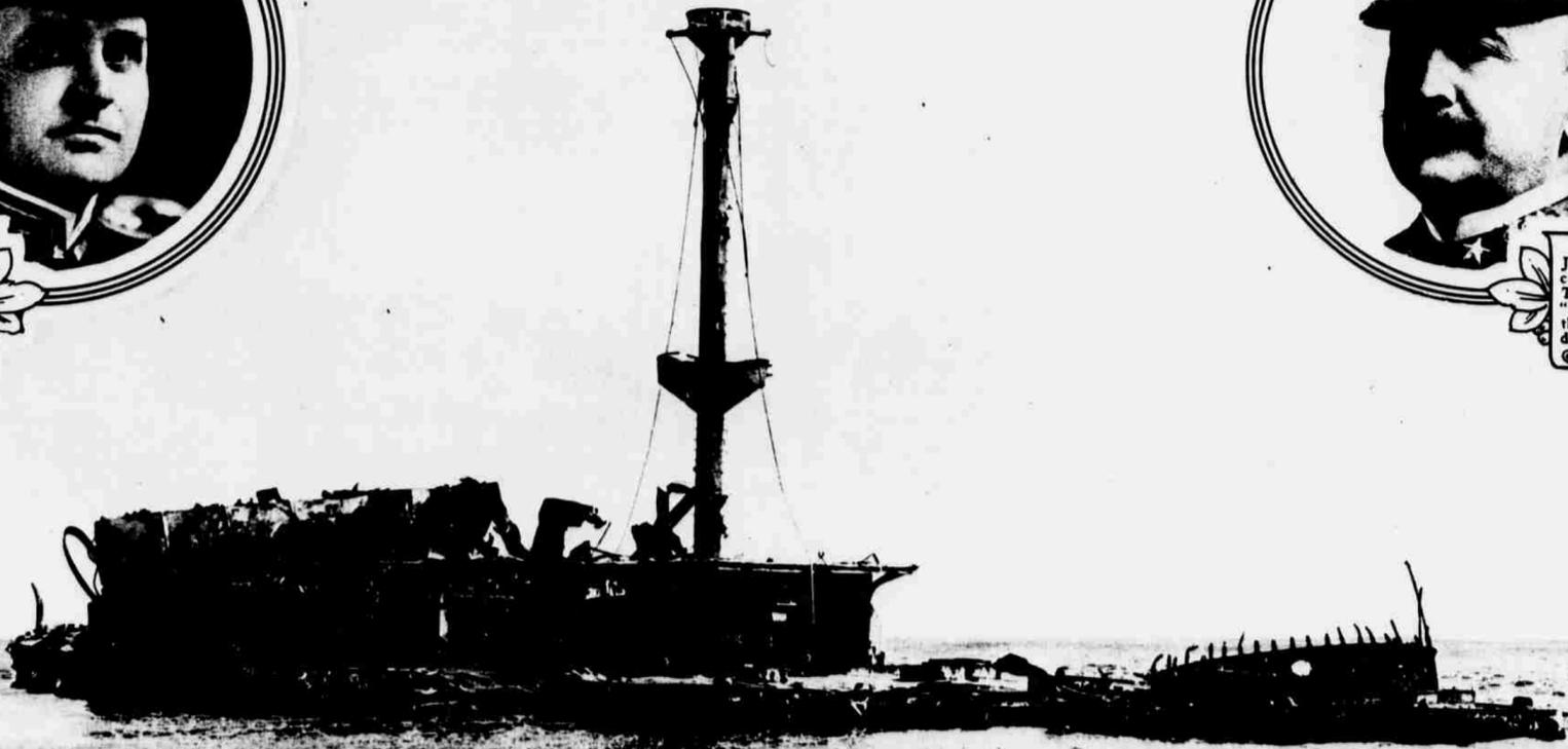
**REMNANTS OF THE OLD TEXAS, TARGET USED IN FIRE CONTROL TESTS OF THE NEW NAVY. NOTE THE OLD MILITARY MAST, THOUGH RIDDLED BY SHELL FIRE, STILL IS STANDING, WHILE AT THE RIGHT THE BASE ONLY OF ONE OF THE NEW BASKET MASTS IS LEFT.**
