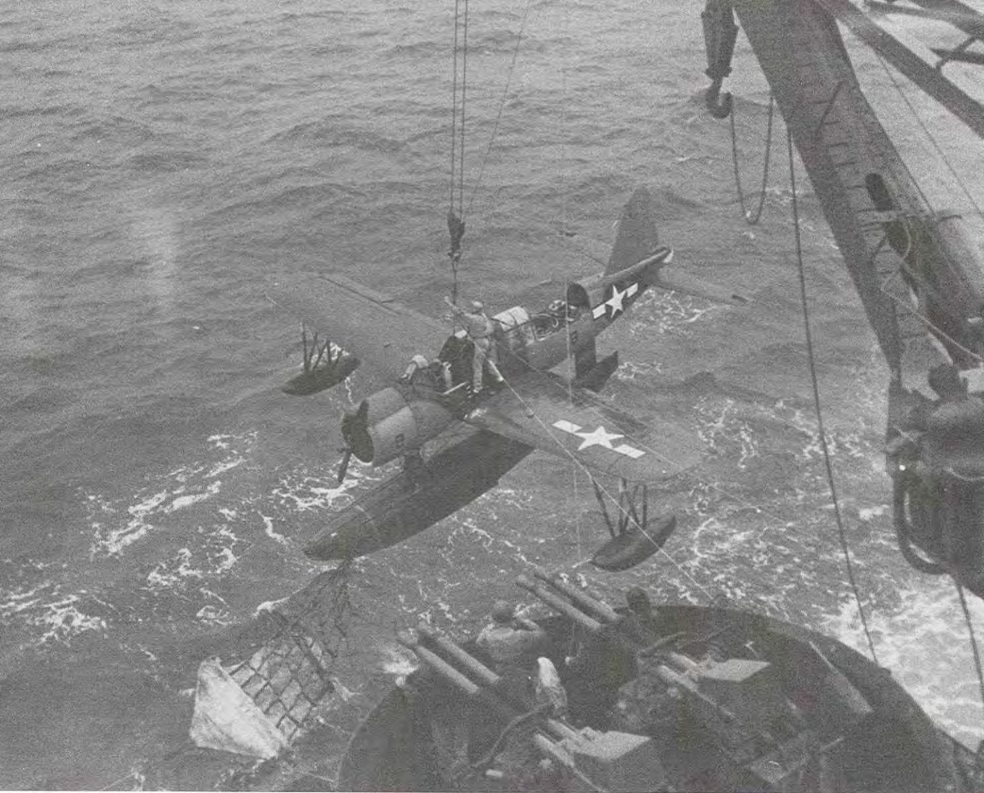
Fig. 20. An OS2U Kingfisher is lifted from the water by Texas ' starboard crane after the aircraft's return from a scouting mission over Iwo Jima on February 16, 1945. One of the aircraft's crewmen attaches lines used to guide the plane as it is moved back to the catapult on No. 3 gun turret. Courtesy National Archives
