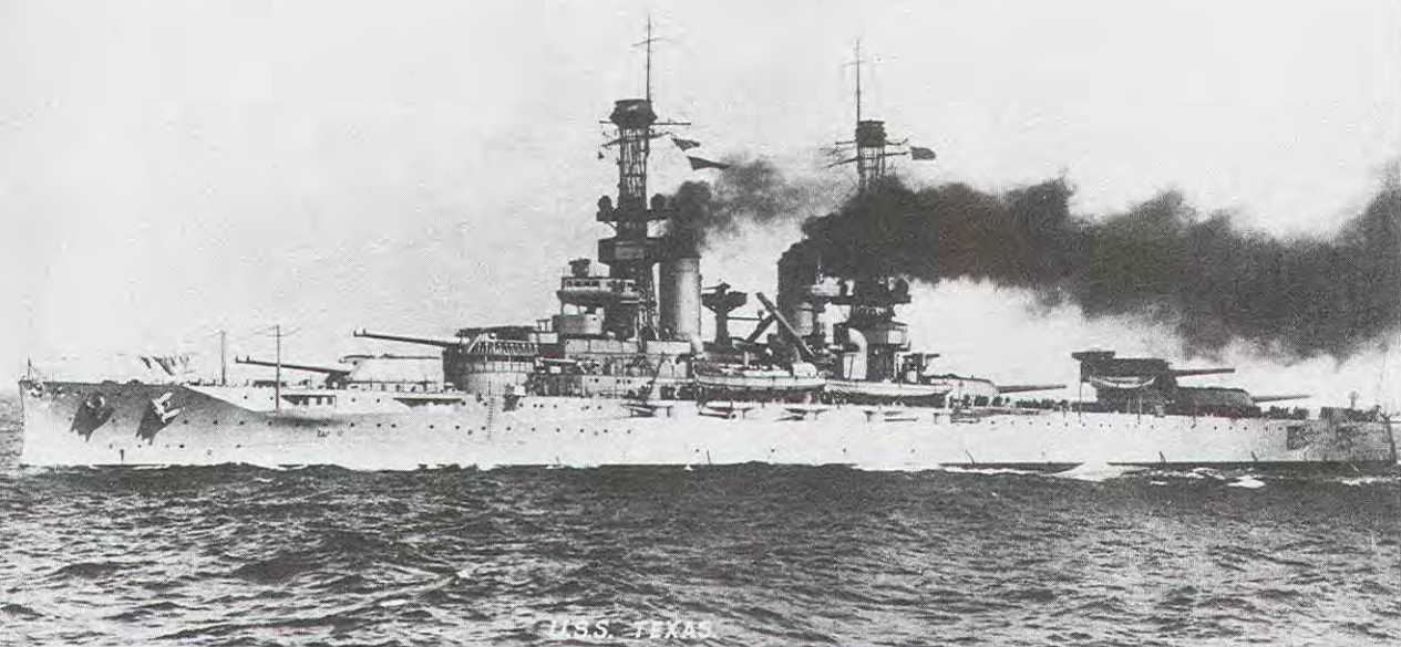
Fig. 25. After World War I Texas showed modifications based on its experience in the North Sea. Here the forward 5-inch guns have been removed and their ports sealed, and an enclosed navigation bridge as well as secondary-battery fire control stations have been added above the armored conning tower. Also note that the optical rangefinders have been reduced to two, located on the roof of the bridge and just aft of the mainmast. Courtesy of The Mariners Museum, Newport News, Virginia
