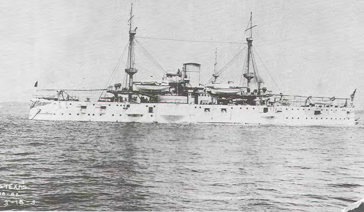
Fig. 22. The first battleship Texas (commissioned in 1895) was short in relation to its beam. The forward 12-inch turret, seen here, is sponsoned out over the ship's port side. The after turret was similarly "echeloned" out to starboard. Smaller guns were mounted on the deck and in hull casemates, and light guns for defense against torpedo boats were carried in the tops. Courtesy U.S. Navy
