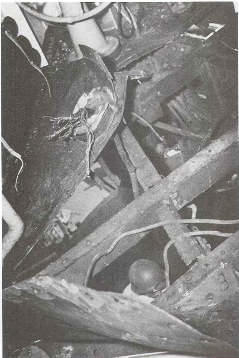
Fig. 16. Texas sustained its heaviest damage during the exchange with German shore batteries at Cherbourg when a large shell hit the armored conning tower and exploded under the navigation bridge. This photograph shows the damage to the floor of the bridge. The base of the helm, the ship's main steering wheel, can be seen at the top of the picture. Courtesy National Archives
