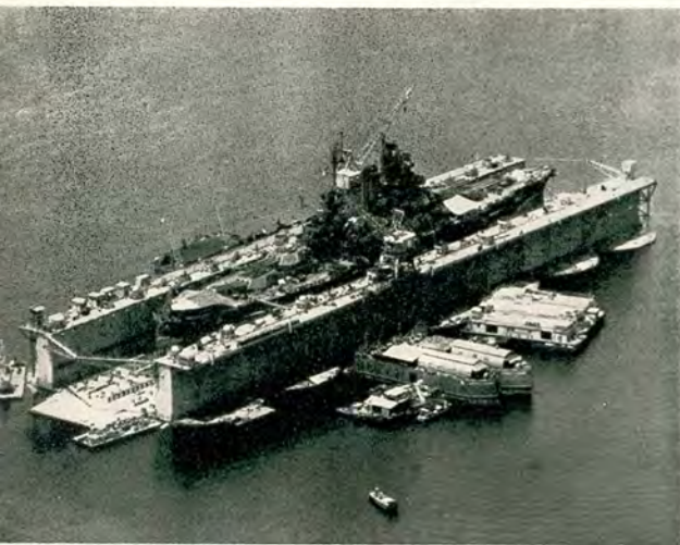
Our battle damage was repaired
