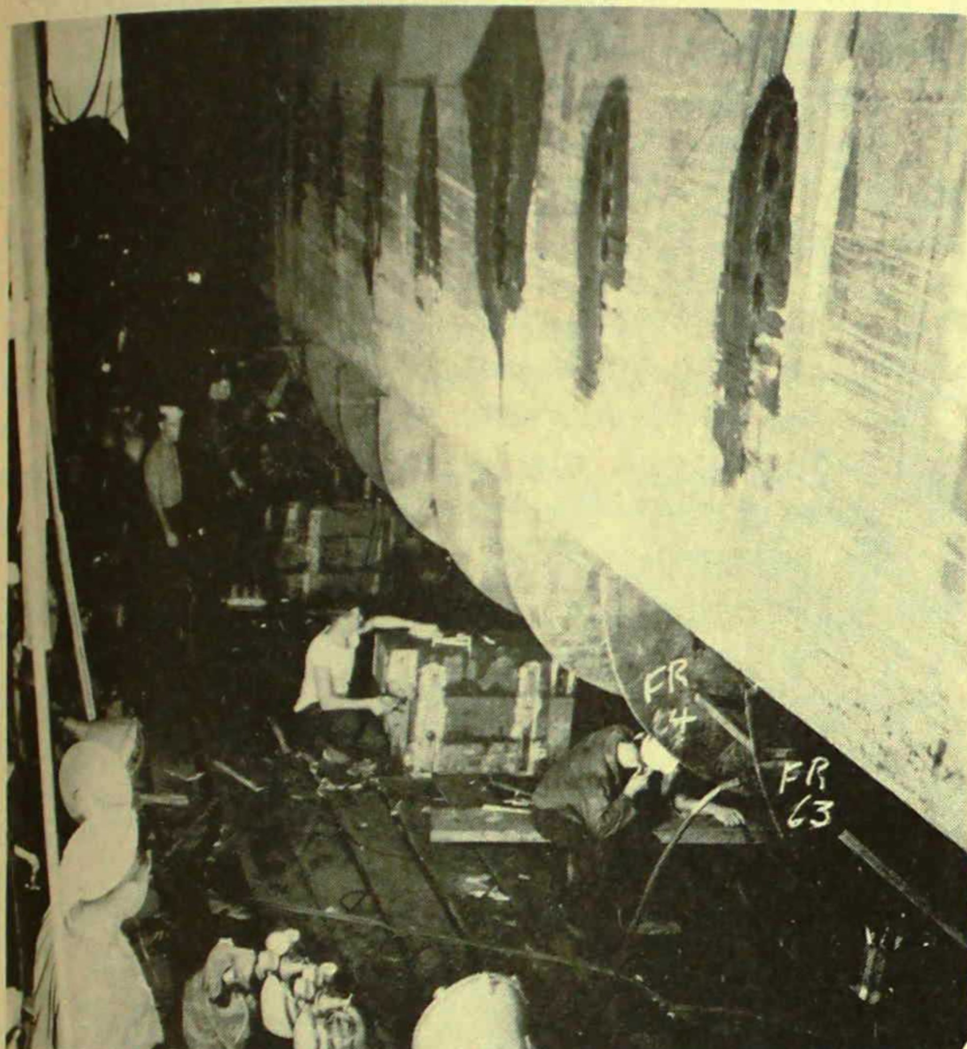
Looking aft, showing faired-in frames
