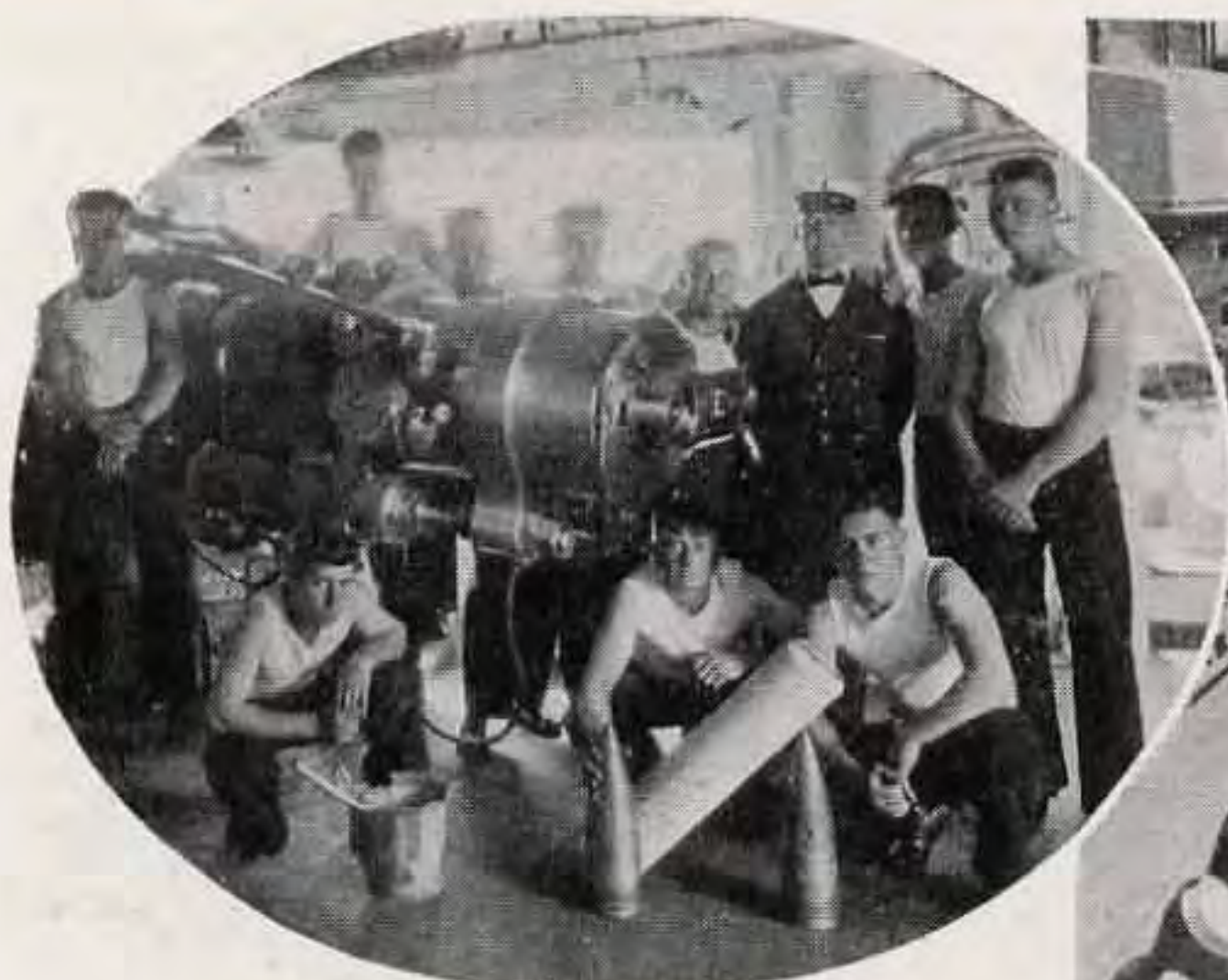
Crew of five-inch gun
