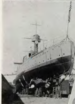
Above—Attaching propellers and painting bottom
