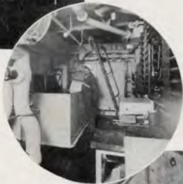
Evaporating plant—for making fresh water from sea water
