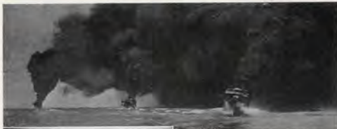
Smoke screen laid down by destroyers as seen from quarter-deck of California
