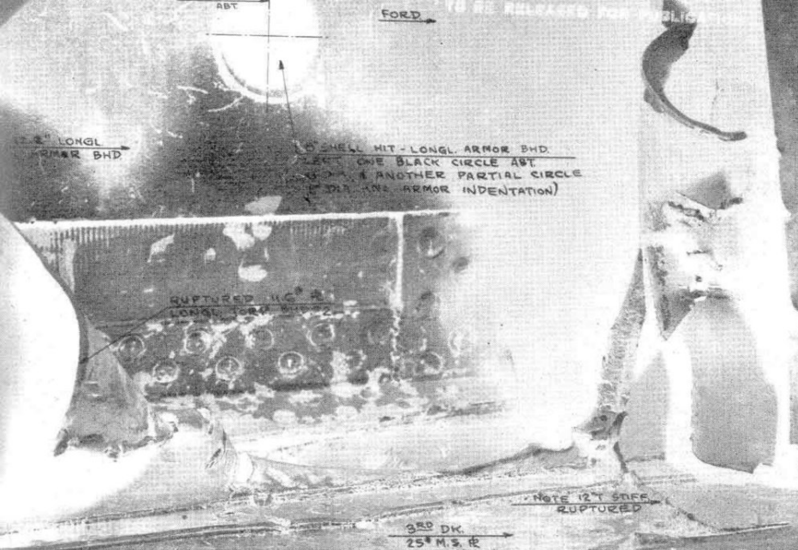
Photo 4: Hit No. 4. Looking inboard through hole in torpedo bulkhead No. 2 to the 12.2-inch longitudinal armor bulkhead. Note mark on armor left by projectile, third deck blown down and torpedo bulkhead blown outboard.
