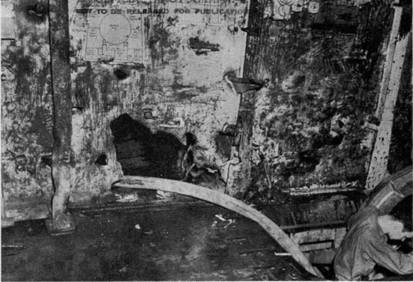
Photo 37: Hit No. 26. Damage to bulkhead 129 above second deck.
