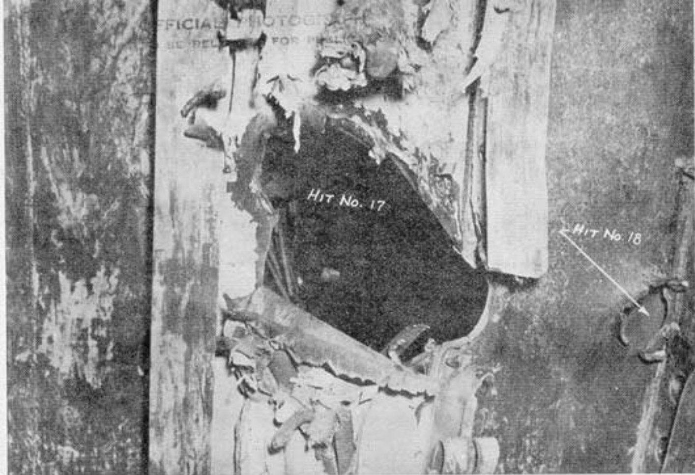
Photo 25: Hits Nos. 17 and 18 on structural bulkhead 9 feet to starboard of centerline.
