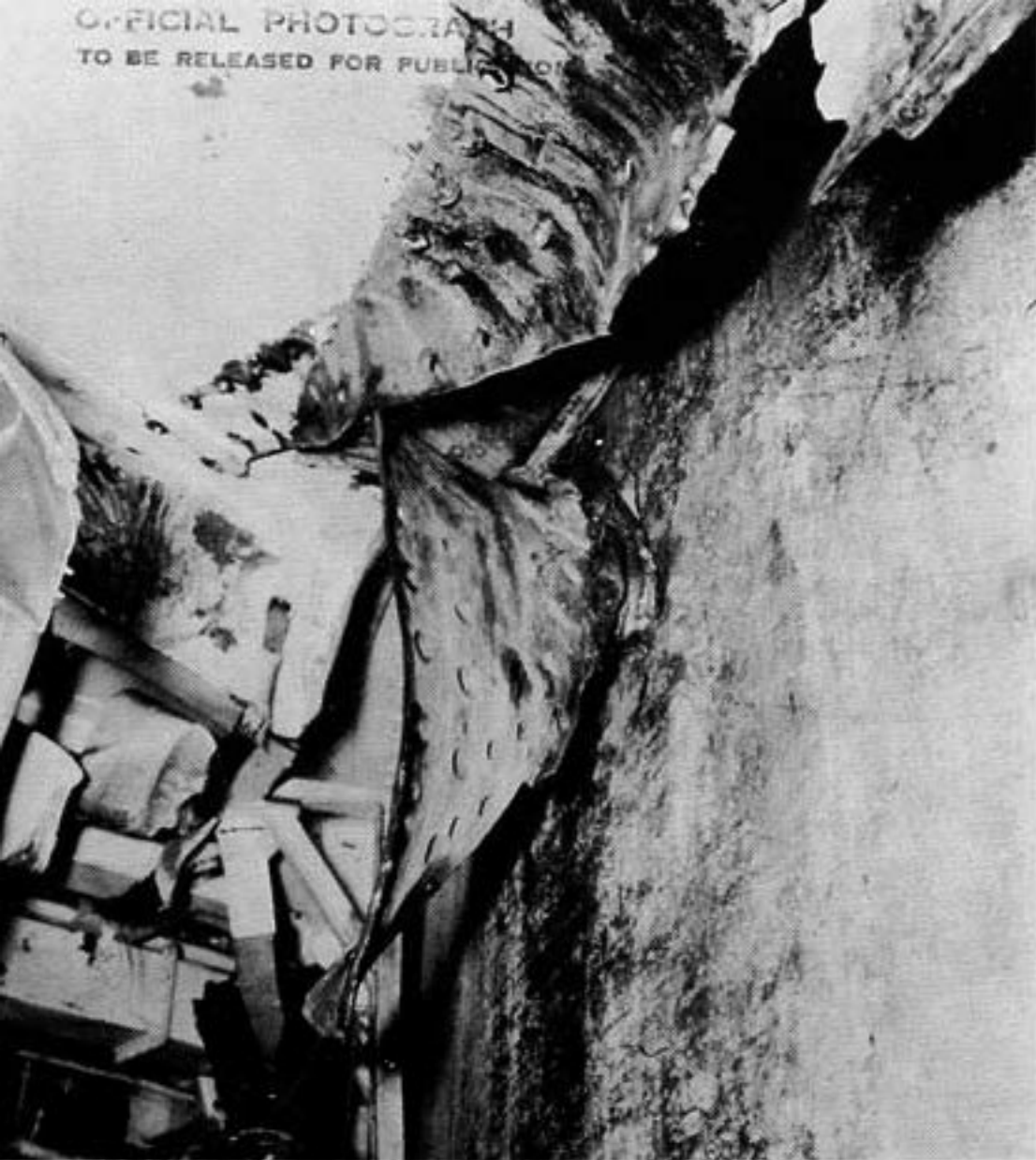
Photo 36: Hit No. 26. Damage to main deck around barbette.
