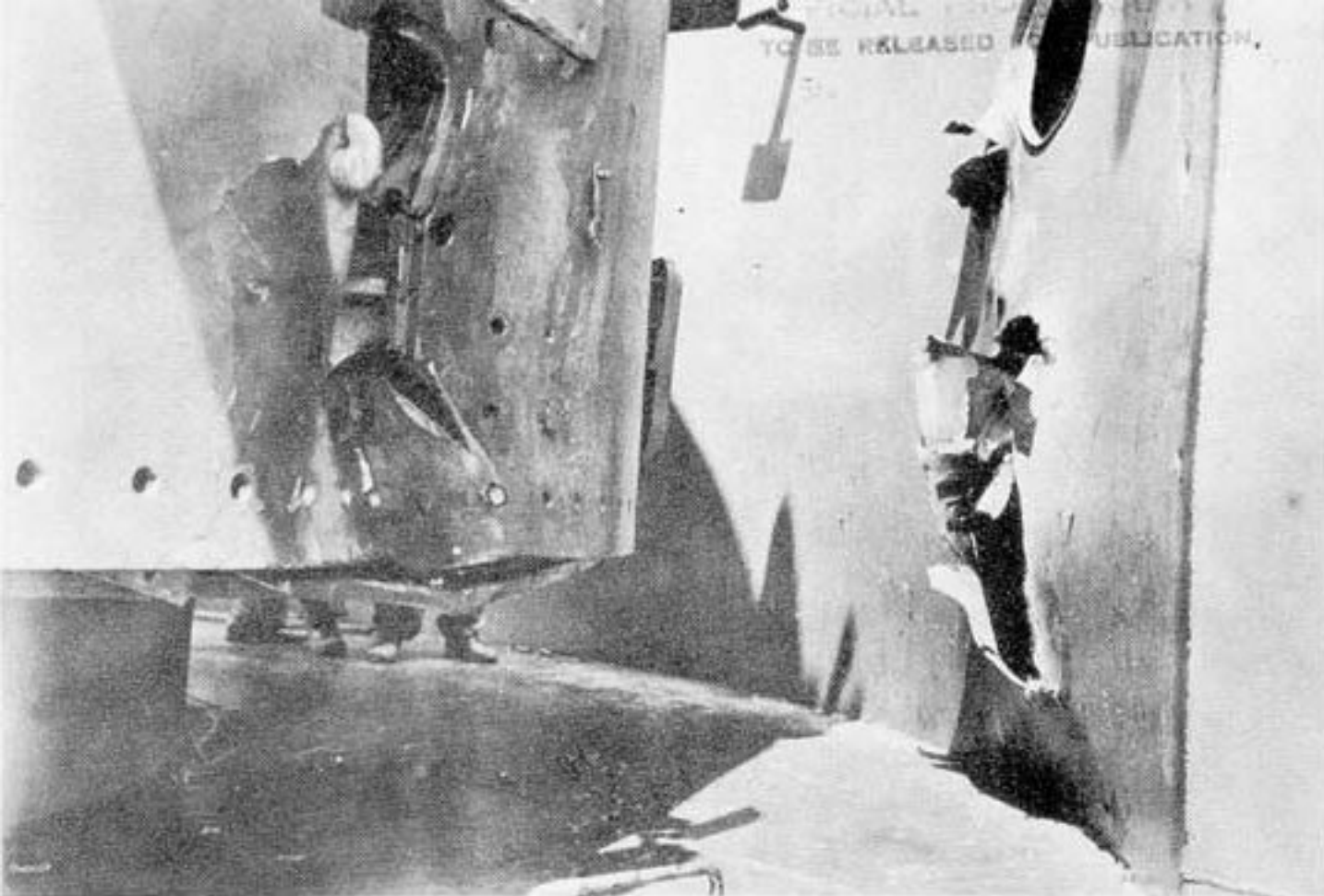
Photo 27: Hit No. 17. Port longitudinal structural bulkhead. Note damage to 5-inch mount No. 2 which stopped this projectile.
