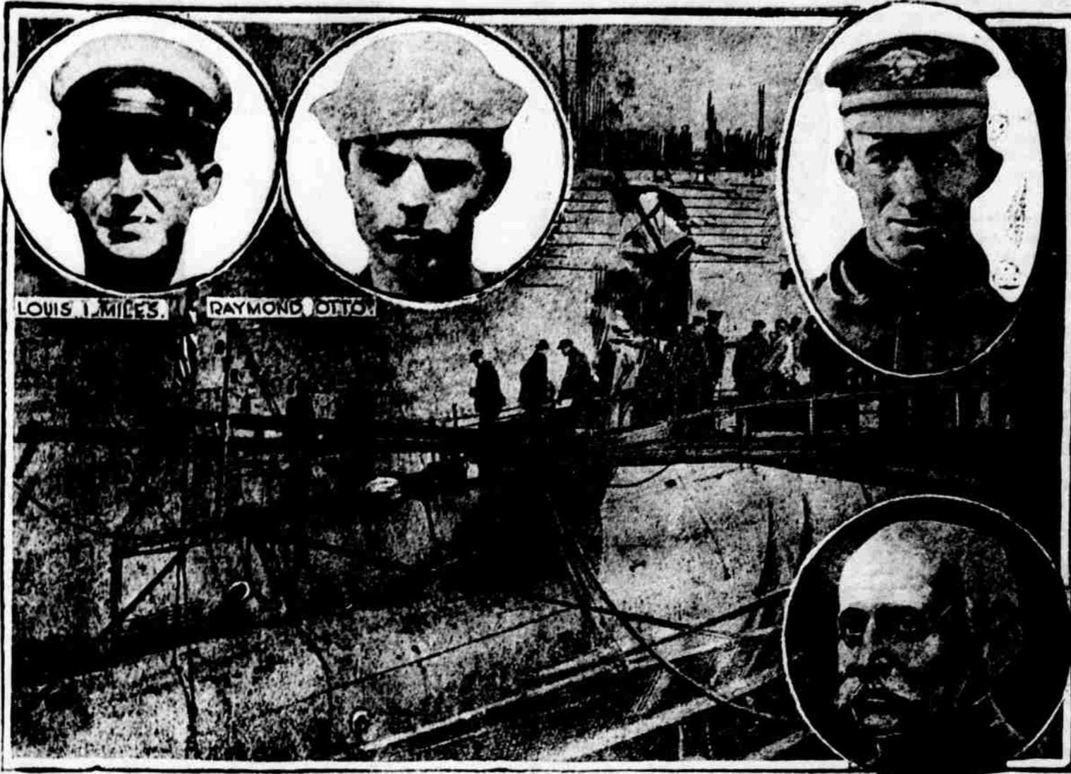
Four men were killed and several more injured when a strange explosion occurred on the submarine E-2 while she was in drydock in the Brooklyn navy yard. Whether the cause was some outside agency or a defect in the machinery of the vessel, or a clunder of a member of the crew, will not be determined without a court of inquiry. Joseph was among those instantly killed. Louis Miles and Raymond Otto, both members of the crew, were seriously injured. Lieutenant Charles M. Cook Jr. was in command of the vessel.
