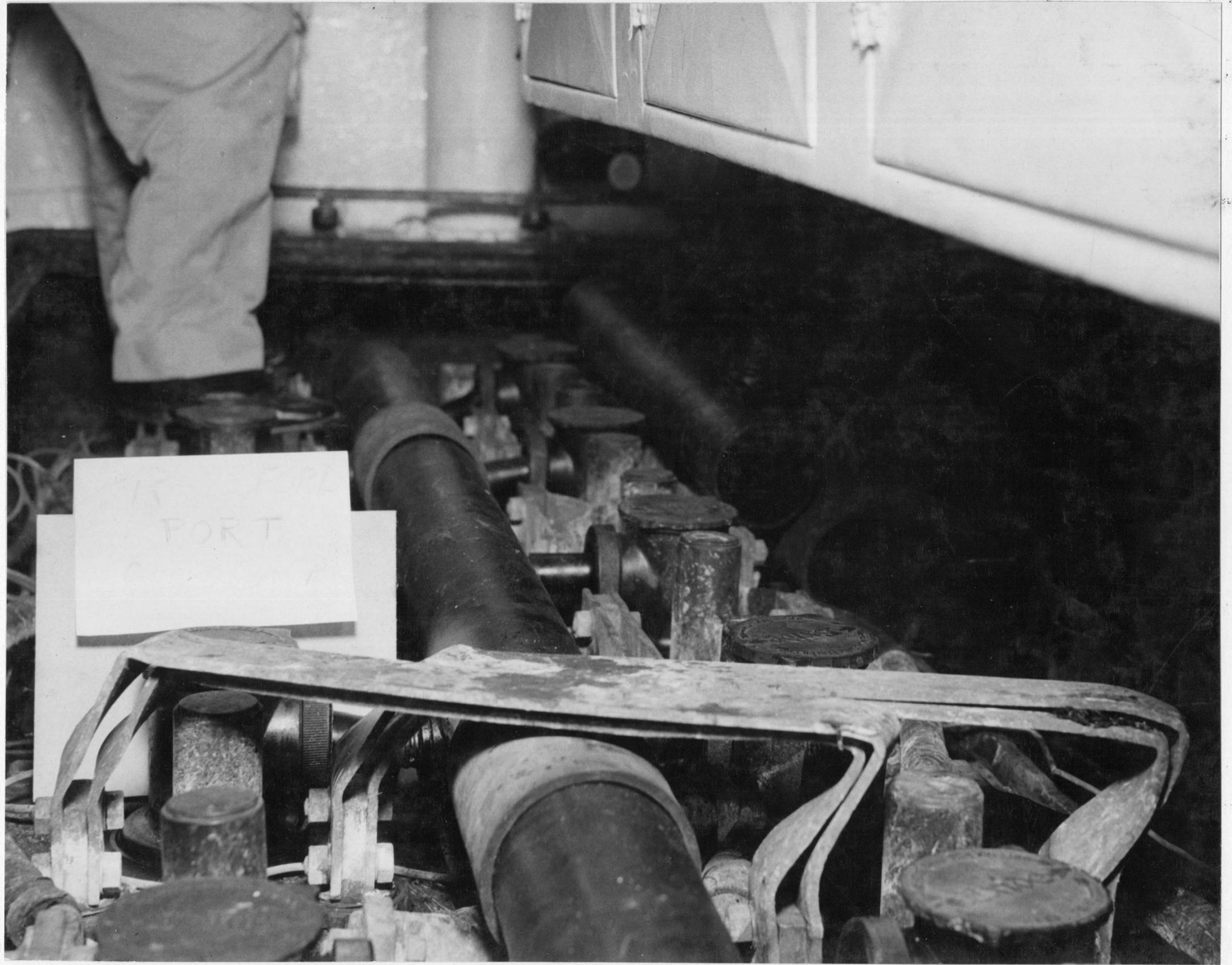
Battery connections for submarine, USS R-2.
