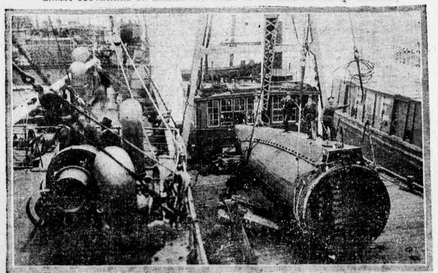
A German mine laying submarine that was captured by the British while laying deadly mines of the coast of England. It was brought to the United States for the purpose of speeding up the second Liberty Loan. This shows a section of the U-boat being raised from the water. It is a heavy piece of work and huge derricks are required.
