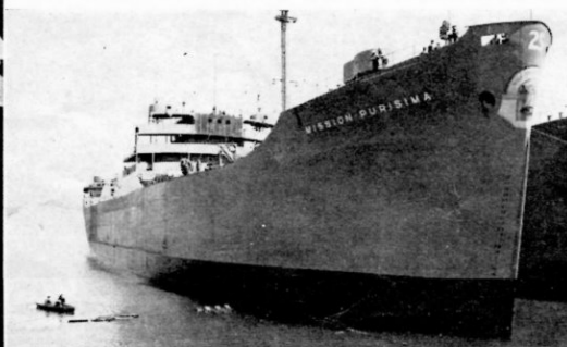
Within a few minutes after launching, the "Purisima" (Hull 25) was warped into outfitting dock and work continued without letup to bring her to a high standard of completion.
