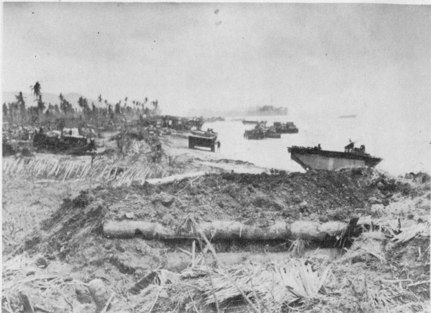
Japanese pillbox set to enfilade the beach; anti-personnel barriers and unloading operations in the background.
