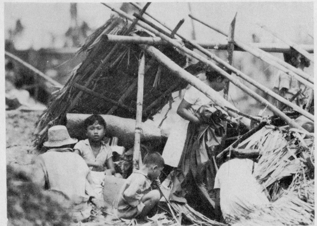
Everything possible was salvaged from demolished homes.
