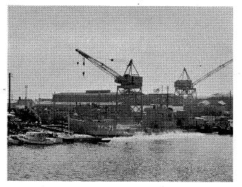
NEW VESSEL LAUNCHED—This unusual side launch of the YFU 71 (Yard Frigate Utility) was necessitated by the narrowness of the channel at Alameda where the ship was built by Pacific Coast Engineering Co. Constructed under the auspices of SupShip 12, the new class of Navy vessel is armed and will be used as a tanker, towboat and freighter in Vietnam.
