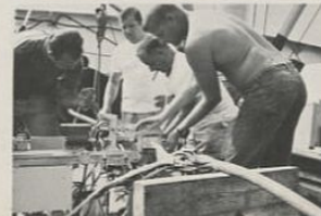
Splicing broken ends of cable. Technicians machine-mold insulation using a heating process. The device on board vessel is called cable jointing machine.
